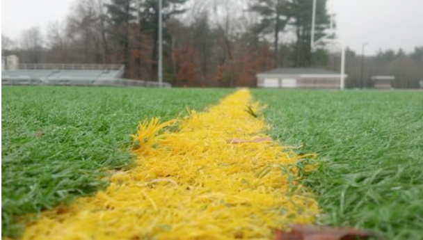
Uneven transition at worn colored fibers
