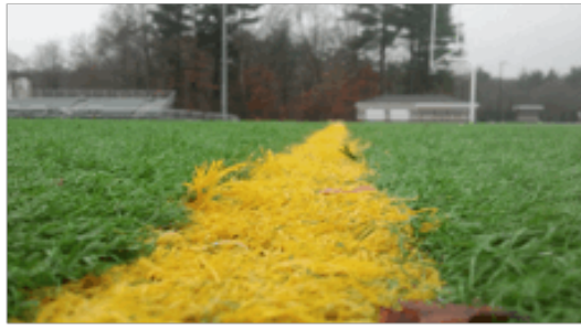
Uneven transition at worn colored fibers Shedding of white, yellow and green fibers throughout
